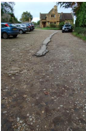
Figure 26: Road surface at Churchfields
