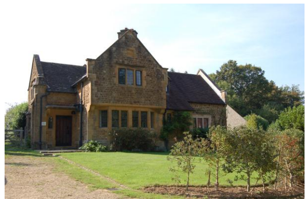
Figure 18: Witley Lodge, Churchfields
