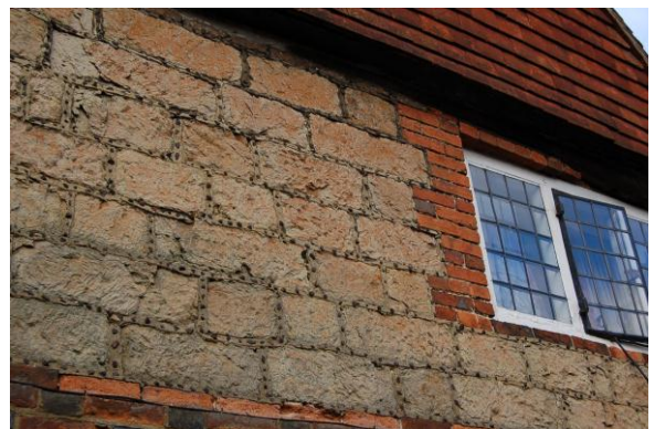
Figure 12: Photograph of the architectural technique 'galletting'
